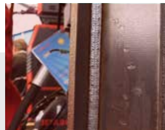
Vertical-up welding without weaving
